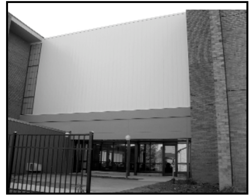
Newly constructed rear walkway connecting the C and B Buildings in Covenant House I.
